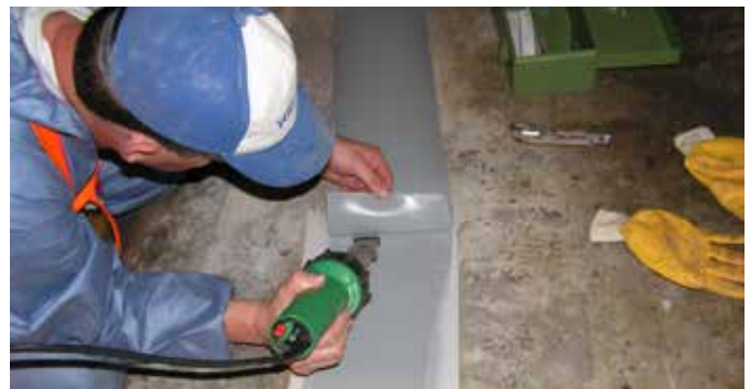
Hot welding butt joints of VANDEX FLEXTAPE
