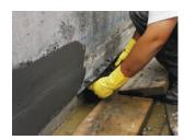
1. Apply a first coat of VANDEX BB 75 E (minimum layer thickness is 2,0 mm, mixing instructions as per Data Sheet VANDEX BB 75 E), at least 1 cm beyond the VANDEX CONSTRUCTION JOINT TAPE.
