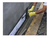
2. Immediately place the VANDEX CONSTRUCTION JOINT TAPE in the freshly applied VANDEX BB 75 E coat. Then, embed both fabric edges in the VANDEX BB 75 E mix.
